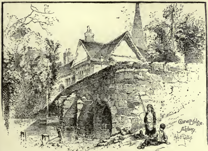
Crane Bridge, Salisbury.
